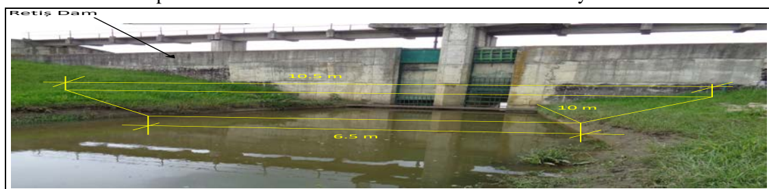
Figure 1: Positioning of the earth dyke – representative scheme.
